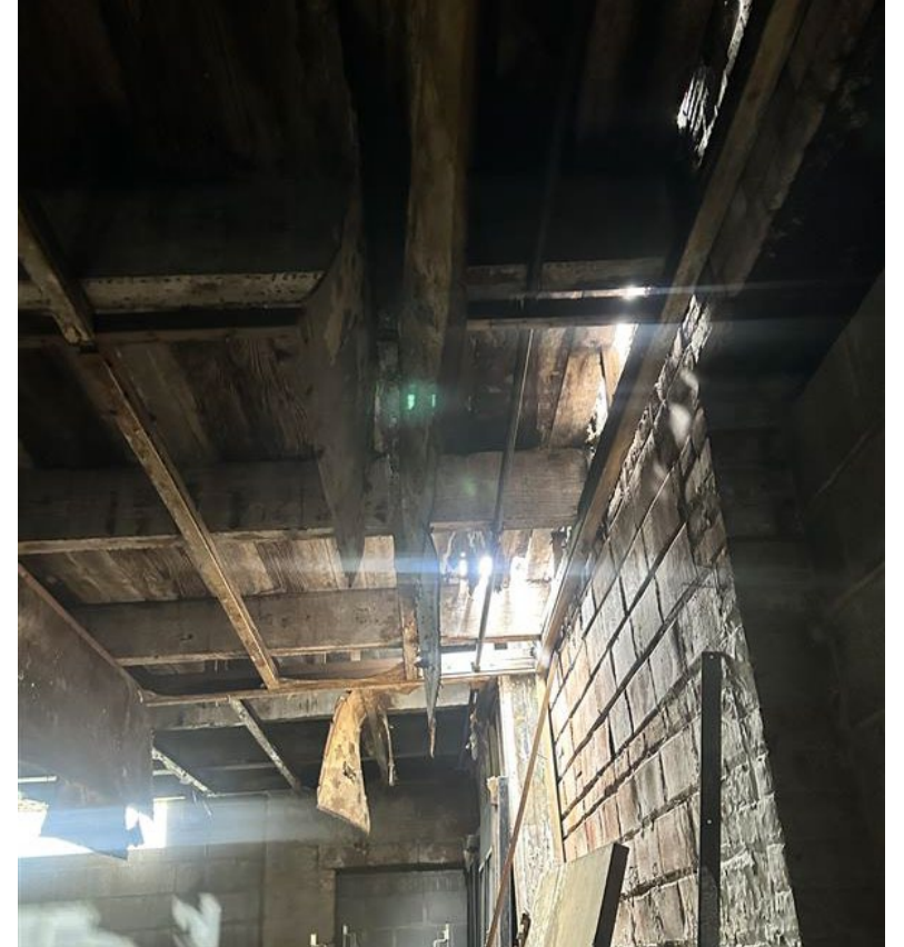
Warehouse & Garage: 2 nd Floor: Rotted and damaged structure
