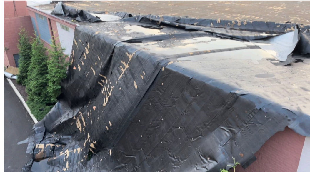
Damage Immediately After Tornado: East Elevation
