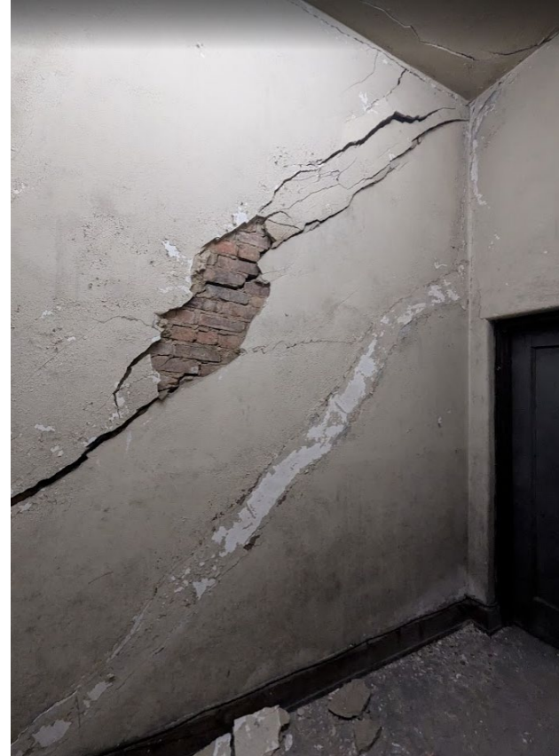
Office & Showroom: 1 st Floor Hallway Significant diagonal step crack visible in masonry wall
