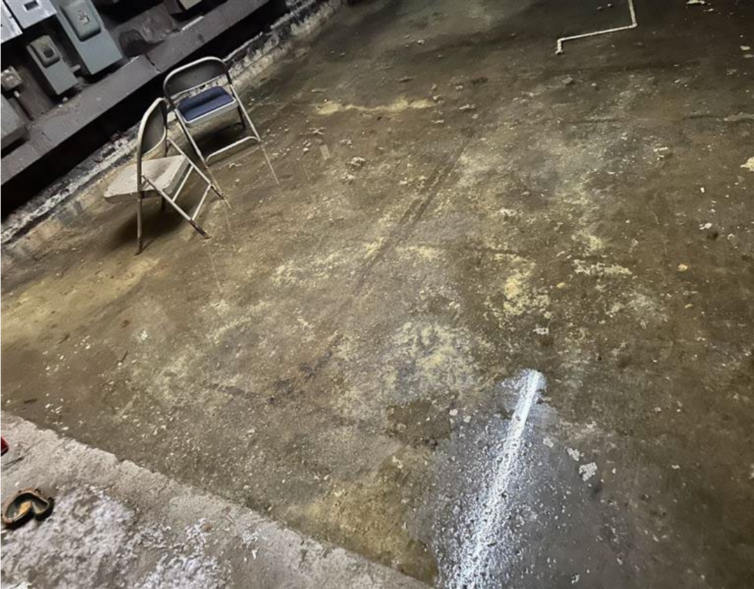
Office & Showroom: Basement with 2-3 inches of standing water
